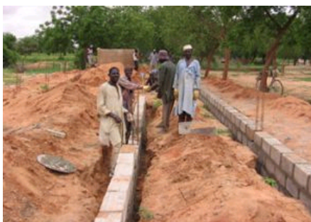
Construction of the new Fistula Centre - Danja, Niger
